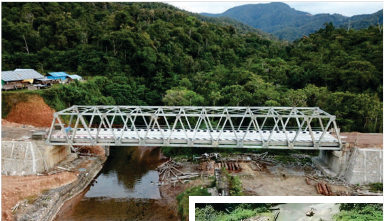
Project Name : Jembatan Rangka Baja A-40 Distance : 40 meter Location : Tekai, Papua Year : 2019
